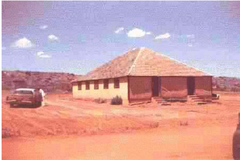
cr03 - The tabernacle with its wood shingle roof, as it looked in the 1970s.
