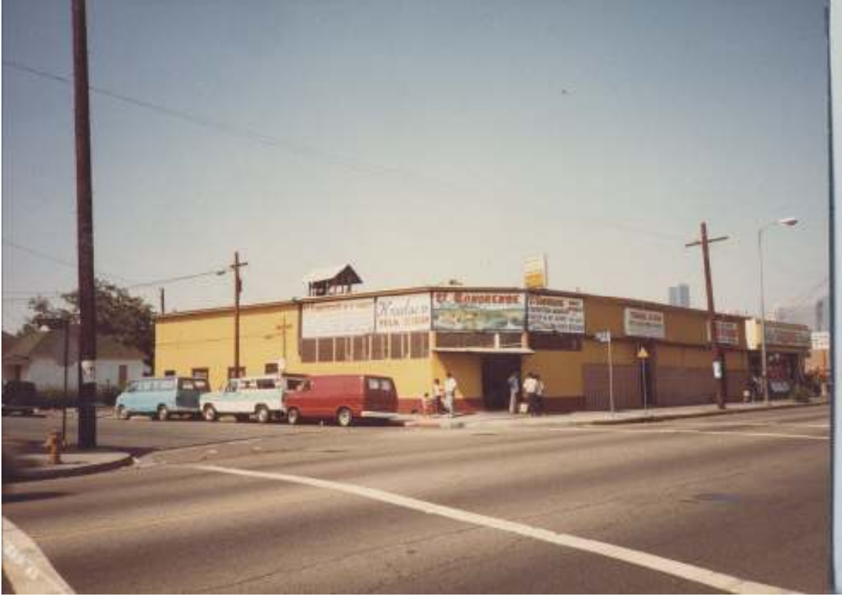
This is the overall picture of the whole store building on the corner of 21 st and South San Pedro Street, Los Angeles
